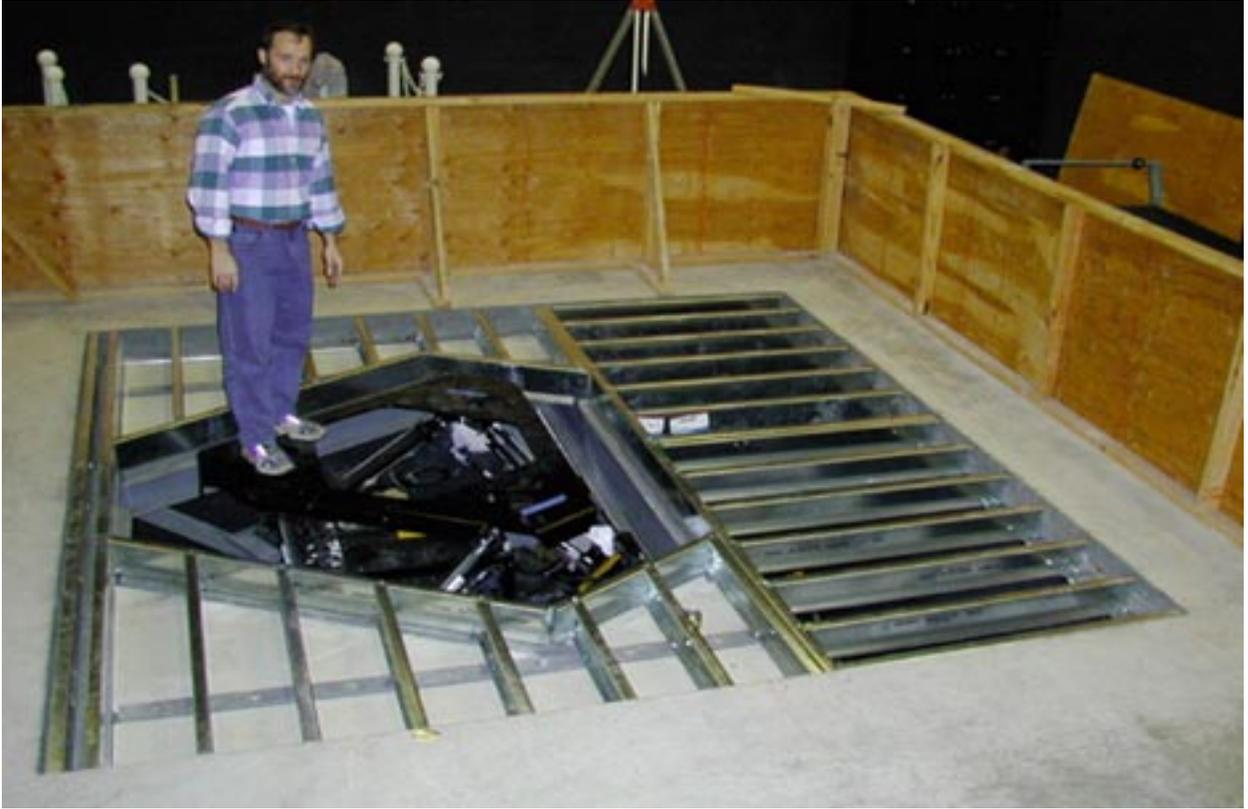
Figure 4. CAVE floor substructure and motion base under construction, February 13, 2001.
